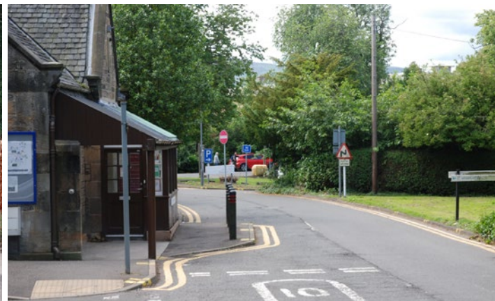
Tipperlin Road entrance - the gatehouse is not in use however does display a noticeboard which provides a route map which is useful to visitors arriving on foot. There is no overall mapping / site plan for drivers arriving on the hospital grounds, so it is difficult to orientate building layout and car parking locations. The pavement is narrow and difficult for wheeled access to navigate.
