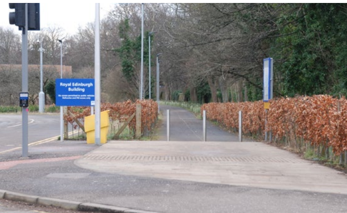
Myreside Road entrance - marked with a change in paving material, streetscape furniture such as lighting, signage and information panel.
