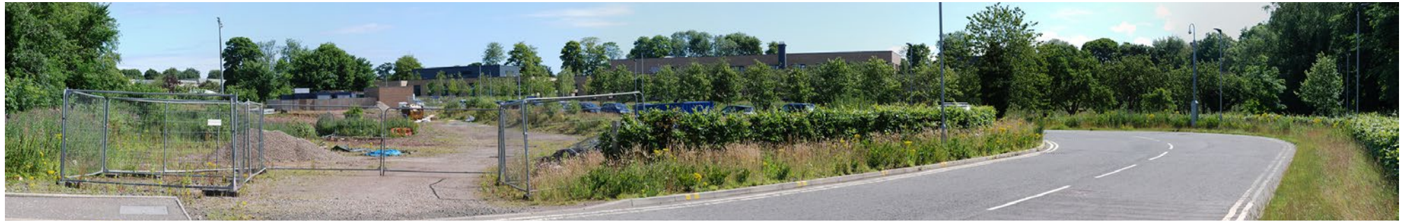
AREA UNDER CONSTRUCTION; REAR (SERVICE ONLY) ENTRANCE TO NEW ROYAL EDINBURGH BUILDING
